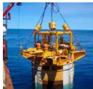
Installation of riser.
