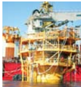
Technip Enfield riser column installation: Exmouth, Australia
