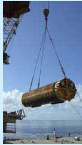
The use of a high-strength, buoyant sling was a must for this stage in the process. The hand-off from the 400-metric-ton overboard crane to the A&R winch was simplified with the help of the AmSteel®Blue grommets. The foundation piles, pump stations, and manifolds were all pre-rigged before the over boarding process.
