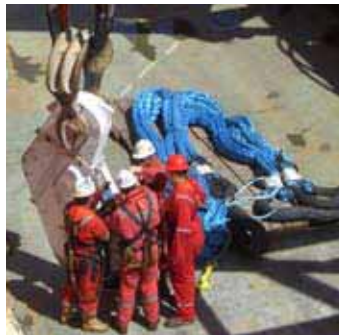
Technip personnel "pre-rig" the hardware packages with the 88-mm AmSteel®Blue grommets.
