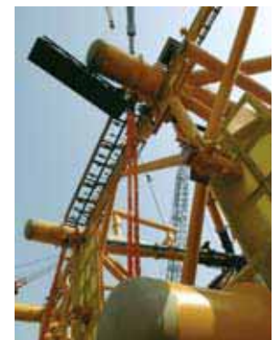
The lightweight, easy handling Quantum-8 slings were attached manually, without the assistance of heavy equipment required by cable-laid or synthetic webbing alternatives, resulting in a faster, more efficient installation.
