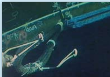
CASCADE AND CHINOOK: ROV handling grommets are used by the ROV to maneuver and position the AmSteel®Blue slings.
