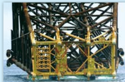
PAN-YU: Quantum-8 high-performance synthetic slings lift 16,213 metric tons.
