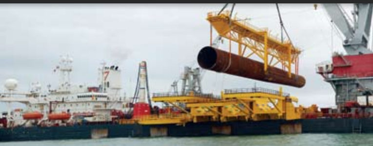
Slings made with Samson's large-diameter AmSteel®Blue lifted 140 monopiles for installation at the Greater Gabbard Windfarm in the North Sea.
