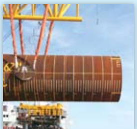
GREATER GABBARD WINDFARM: All 140 turbine foundation monopiles were installed using the first set of lifting slings. After completion Lloyd's proof loaded the slings and recertified them for continued use.
