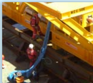
CASCADE AND CHINOOK: ROV handling grommets are used by the ROV to maneuver and position the AmSteel®Blue slings.
