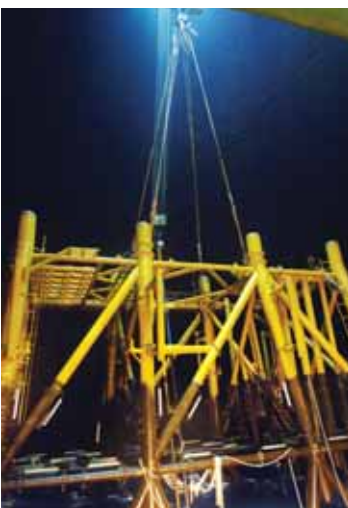
Quantum-8 high-performance synthetic slings lift 16,213 metric tons on COOEC installation. (March 2008)
